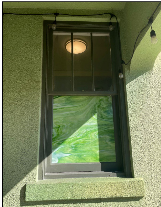
Figure 5: Window to be replaced. Significant deterioration is not visible.
