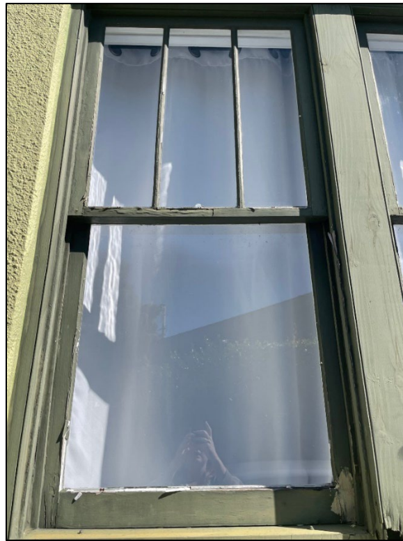
Figure 2: One window proposed to be replaced.
